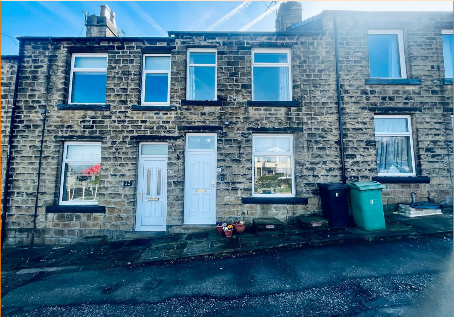
Brick Bank , Huddersfield, HD5 8RU
